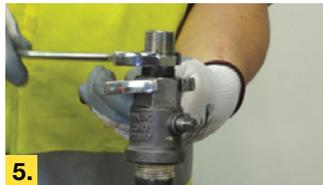
**5.** The Nipple should be tightened until the hexagonal part touches or is within 1mm of the top of the Body. A second spanner or grip will be also required to stop the Body rotating and act as a restraint.
