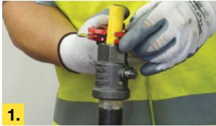
**1.** With the Nipple and Olive removed from the body, cut the PE pipe close to the top of the body or if the PE is movable, pull back the cut end until flush or within 5mm of the top of the Body.
