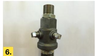
**6.** The fitting is now complete. Attachment of the ECV and pressure testing can now be completed before grouting is commenced following manufacturer's instructions. Once complete the fitting can be finally sealed by replacing the 1/4" Plugs and sealing with suitable thread sealing compound.
