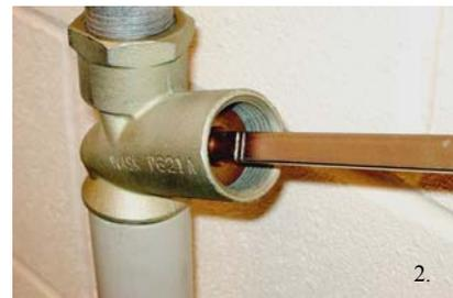
Note:- Do not screw the plug out beyond this point as the closure plug seal will not seat on the fitting body.
