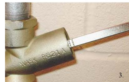
3. Replace the closure plug and tighten firmly using the key pins on the other end of the activation tool.
